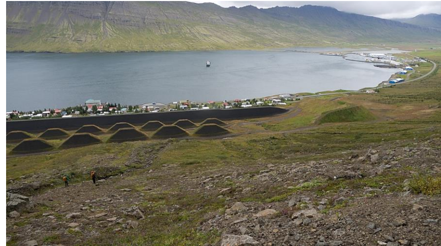
Figure 2. Catching- and deflecting dam below Tröllagil gully in Neskaupstaður, East Iceland.
